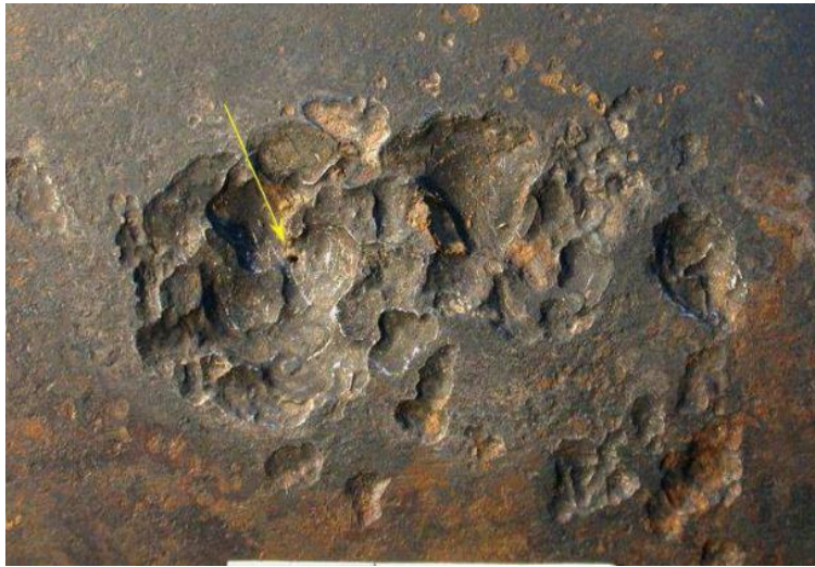
Photo 4.20B. Image of damage as a result of the inductive interaction of a high-voltage line
